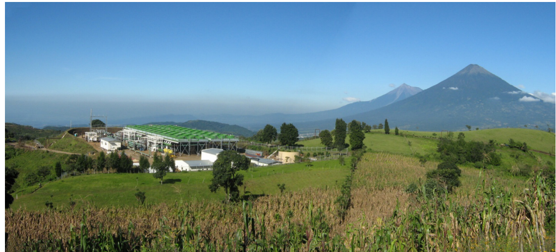
Amatitlan Power Station, Guatemala
